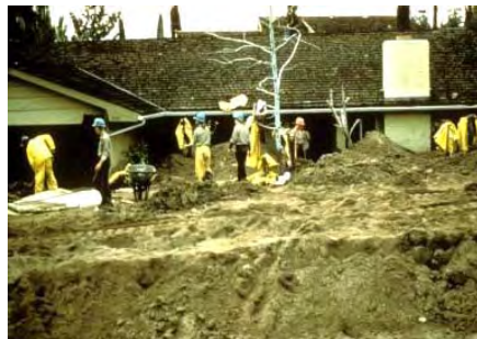
Figure 1 —Post fire erosion problem.
