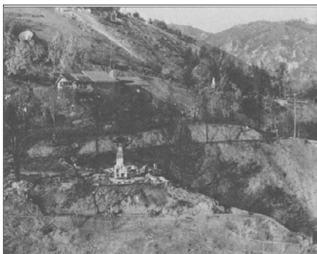
Figure 1 —A home located in upper Las Flores Canyon, Malibu, California, that survived the Old Topanga Fire because of homeowner preparations.
