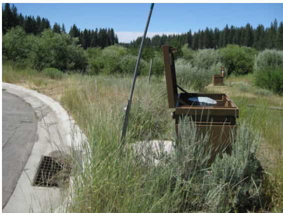
Photo 3: Job boxes housing auto samplers. Foreground: inlet at end of cul-de-sac, background: basin overflow weir.
