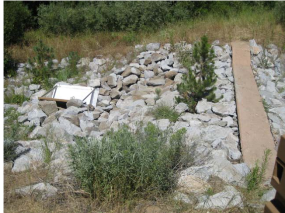
Photo 2: Detention basin concrete overflow weir and flow measuring flume.
