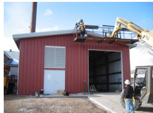
For Schools boiler building in Ely, Nevada, under construction.
