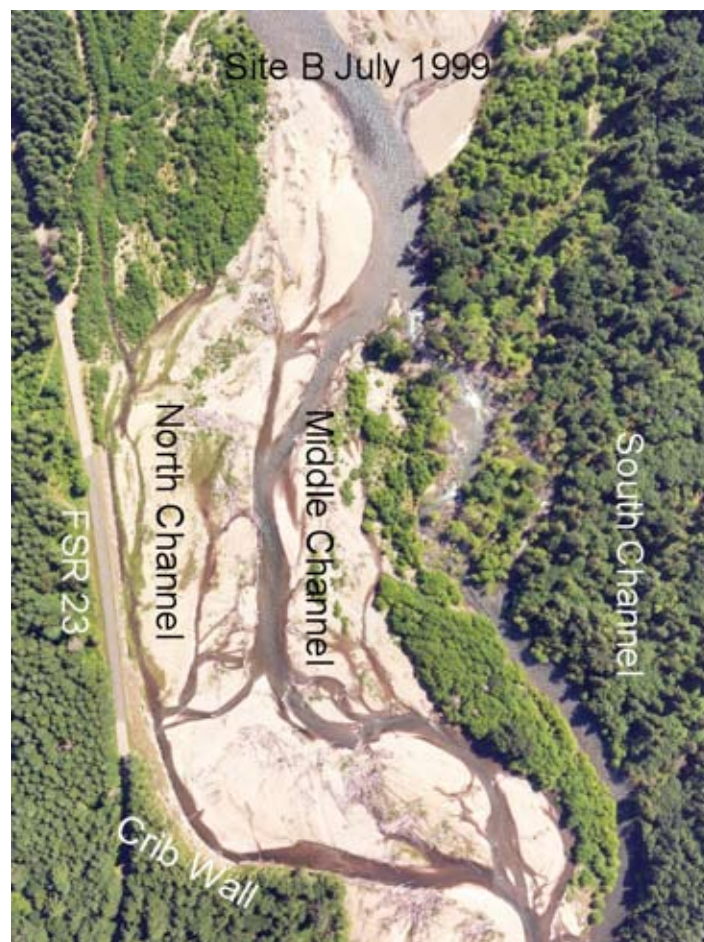
Figure 5 - Site B in 1999, before the construction of the logjams.
