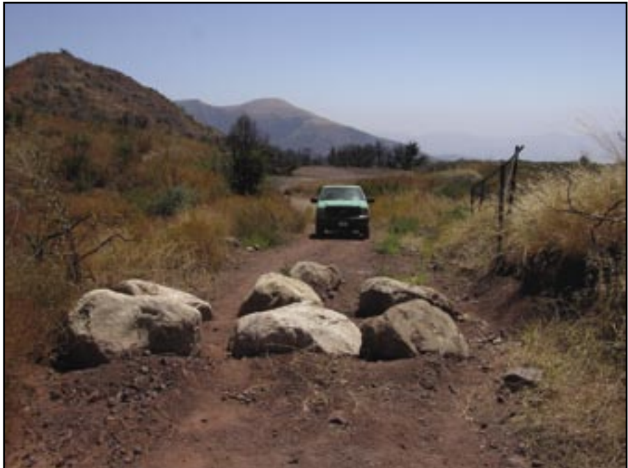
Figure 105—Boulder barricade prevents vehicle entry but allows pedestrian access.
