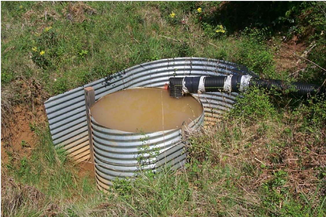
Figure 4 Ditch inlet structure that collects water and diverts it to the settling basin
