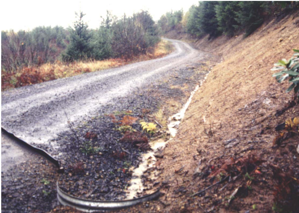
Figure 1. Downslope end of road runoff plot with ditch diversion inlet in foreground for collection pipe.
